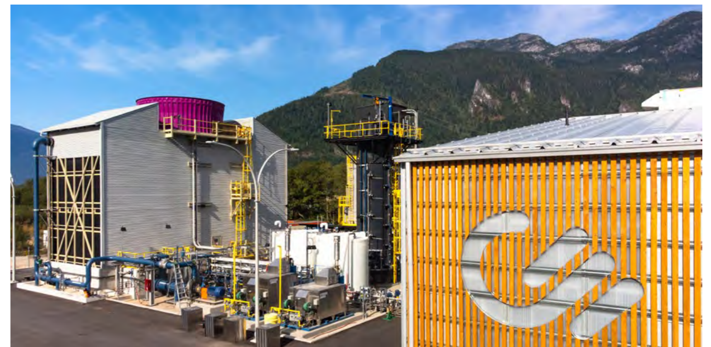
Carbon Engineering's Innovation Centre and Advanced Development Headquarters located in Squamish, Canada.
