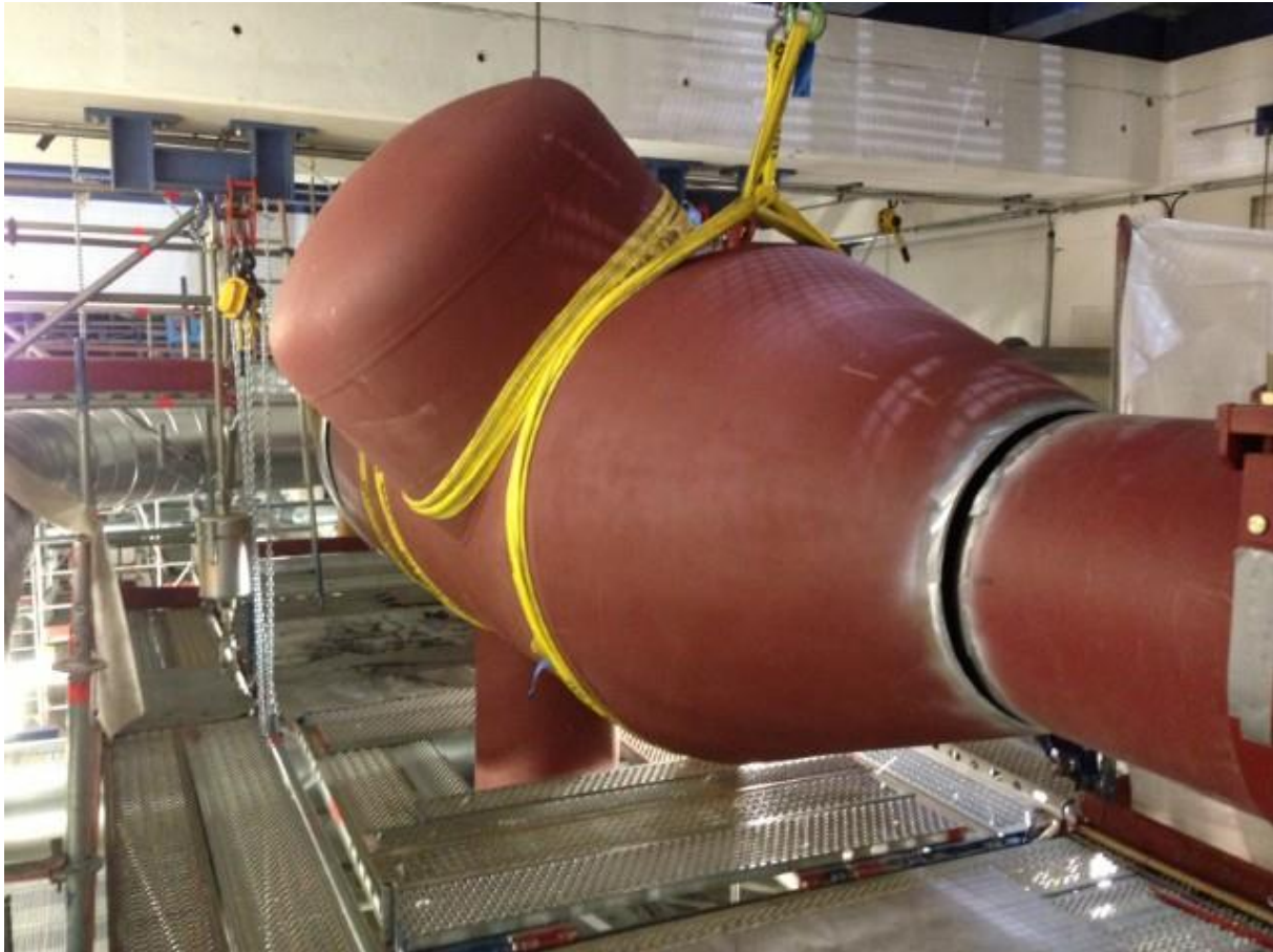
Figure 3.5 View of the the low pressure tie-in piece being mounted (April 2013)
